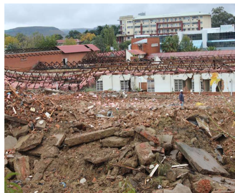
QUEEN Elizabeth II Hospital in Maseru is currently being demolished.
