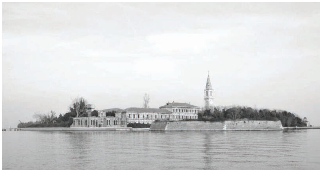
A PHOTOGRAPH showing the only standing buildings on Poveglia Island.
