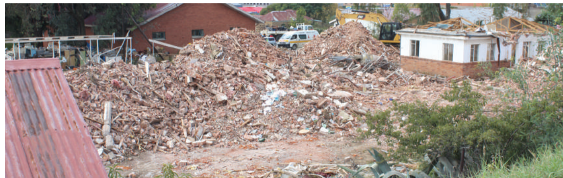
QUEEN Elizabeth II Hospital demolition work is behind schedule.
